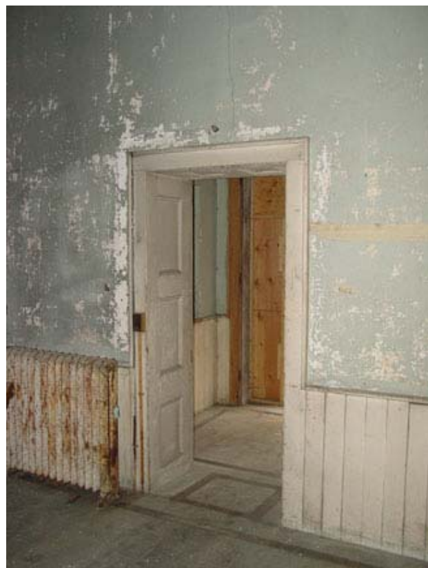
Figures 66, 67 and 68. Details of the Transepts. Above is the decorative screen designed by George Hanley. Note the shoring installed by the National Parks Service below the screen. Lower left, detail of run plaster moldings in west Transept. Lower right, doorway into west Entryway. Note the paneling on the door jam and the wainscoting that wraps around the entire space of the main floor.
