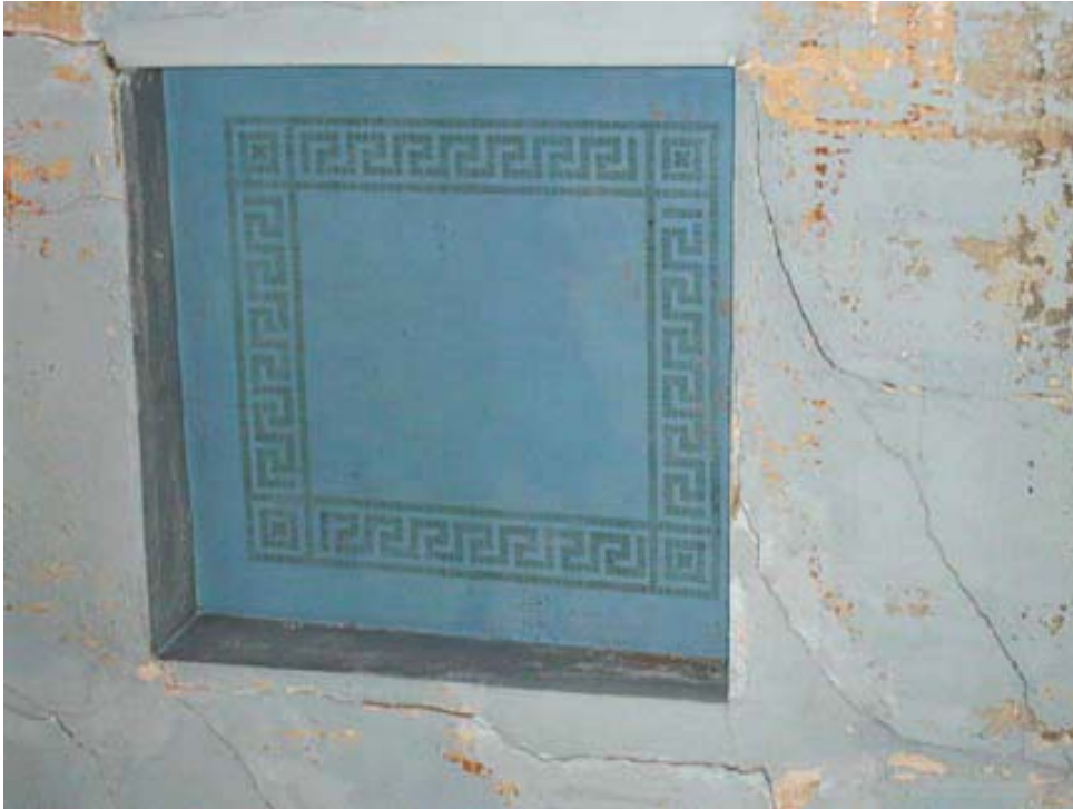
Figure 63. View of ceiling coffer from Nave. The Greek key pattern is visible in all the coffers. The ribs between the coffers are also decorated with stencils.
