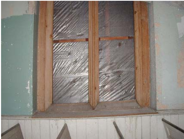
Figures 60 and 61. The existing window frames were installed in 1867-8, reducing the size of the sash by half. (above) The remaining sash were stripped, broken glass removed and then stored in the east Transept.
