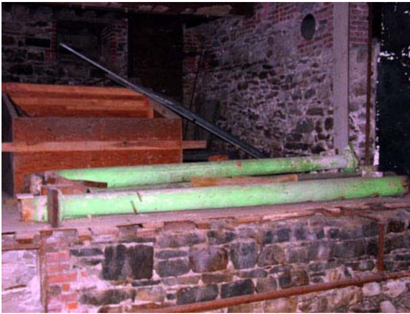
Figure 40. Original wood columns currently stored on basement stage. The columns should be restored and reused in the Sessions Room. The stone wall visible on the right was likely part of the 1860 building campaign that addressed the acoustical problem of the Nave upstairs by creating an apsidal recess and Pastor's Study.
