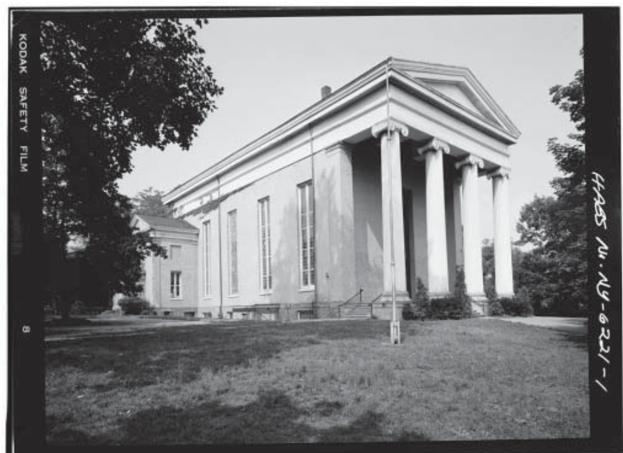
Figure 17. West elevation taken during Historic American Building Survey in 1967.
