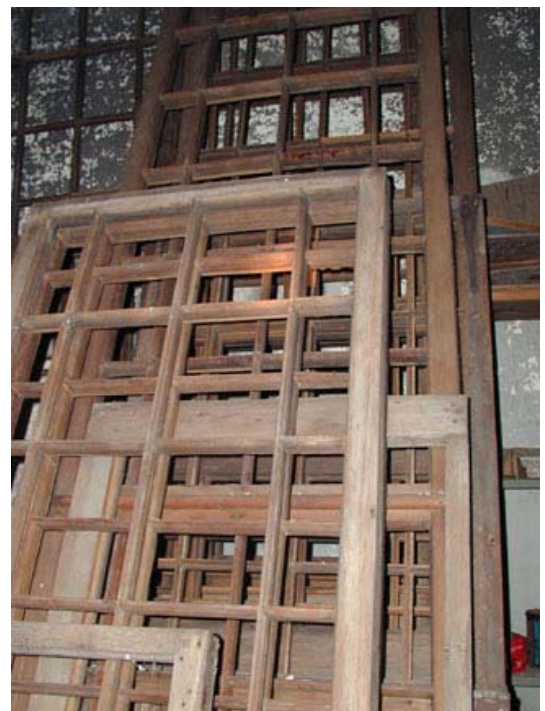
Figures 60 and 61. The existing window frames were installed in 1867-8, reducing the size of the sash by half. (above) The remaining sash were stripped, broken glass removed and then stored in the east Transept.
