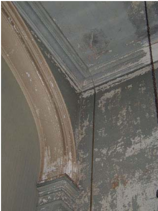
Figures 66, 67 and 68. Details of the Transepts. Above is the decorative screen designed by George Hanley. Note the shoring installed by the National Parks Service below the screen. Lower left, detail of run plaster moldings in west Transept. Lower right, doorway into west Entryway. Note the paneling on the door jam and the wainscoting that wraps around the entire space of the main floor.
