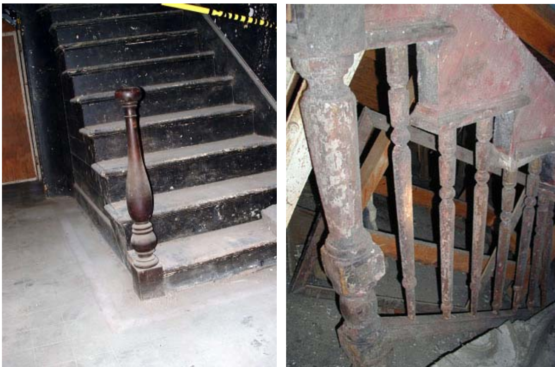
Figure 64 and 65. Stair leading from Vestibule to the east Gallery is original to the building. Remnants of the balusters and rails are stored in the east Transept.
