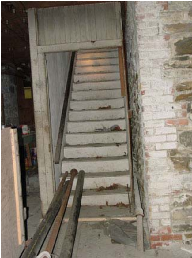
Figure 43. Stairs leading from basement Stage to west Transept as likely added during the 1867-8 alterations. It follows a stone wall constructed after the original building campaign of 1835; its function is unknown. Note the brick masonry used to finish the corner.
