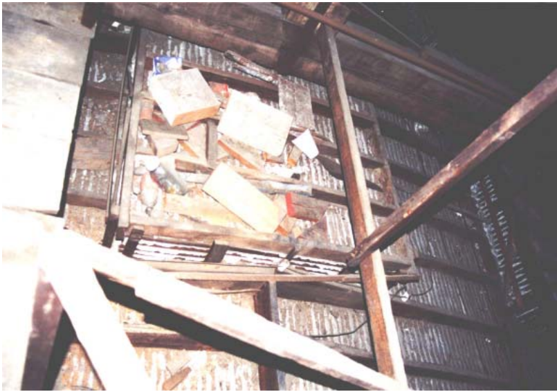
Figure 58. View of ceiling coffer from attic. The ceiling is suspended from the trusses. The coffers are approximately 12" deep.
