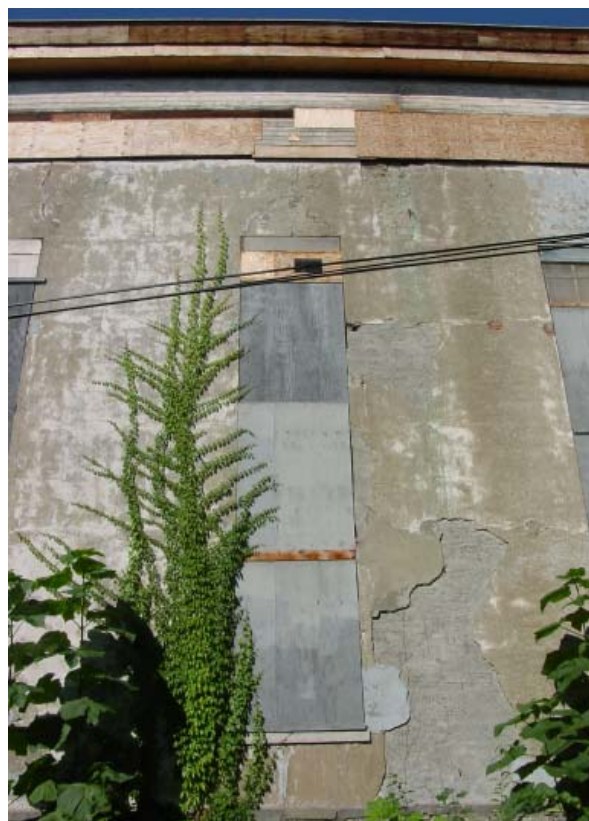
Figure 24. Spalled stucco on east facade between window W23 and W24; note plywood covering portions of entablature.
