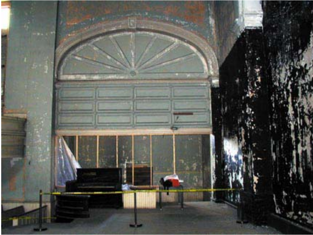
Figures 66, 67 and 68. Details of the Transepts. Above is the decorative screen designed by George Hanley. Note the shoring installed by the National Parks Service below the screen. Lower left, detail of run plaster moldings in west Transept. Lower right, doorway into west Entryway. Note the paneling on the door jam and the wainscoting that wraps around the entire space of the main floor.
