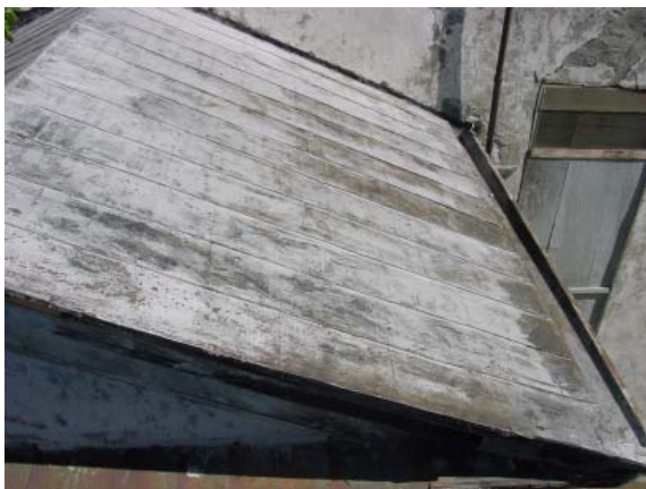
Figures 35 (left) and 36 (above). West entry roof with aluminized coating. Although there is general wear, the roof does not need immediate repair. The roof of the west Transept is a flat seam metal roof very much in need of repair. The roof of the west Transept is standing seam metal. The pans have lost their protective coating and show signs of deterioration which may lead to leaks affecting the interior of the building.
