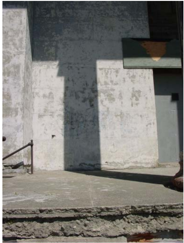
Figure 31. The protected lime rendering on the south wall illustrates the scribed ashlar pattern specified by Davis. Note the holes in and deterioration of the rendering at various locations in the photographs. Later coats of paint are peeling from the surface. Also note the spalling apparent on the concrete deck in the foreground.
