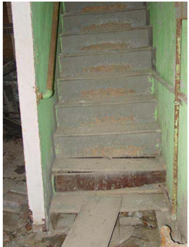
Figure 49. Stairs connecting East School room to vestibule of main level. Communicating stairs between the levels should be installed to facilitate ease of movement through the building.
