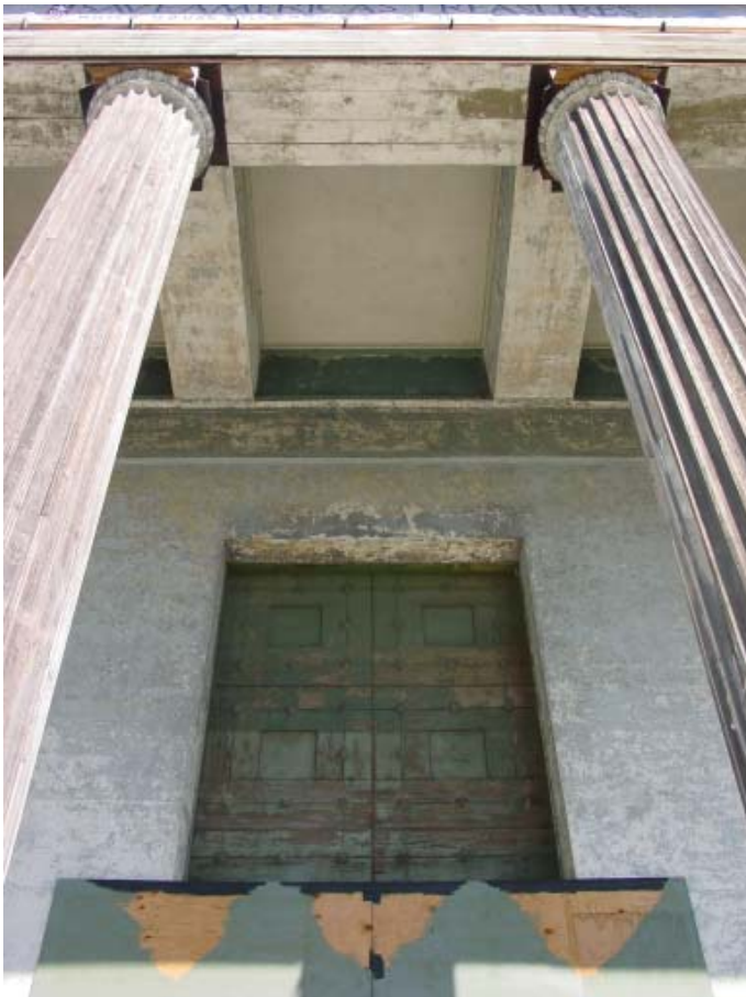
Figure 31. The protected lime rendering on the south wall illustrates the scribed ashlar pattern specified by Davis. Note the holes in and deterioration of the rendering at various locations in the photographs. Later coats of paint are peeling from the surface. Also note the spalling apparent on the concrete deck in the foreground.
