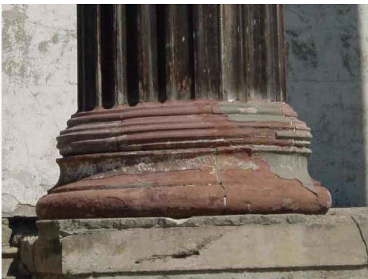
Figures 26 and 27. Base, capital and shaft of Ionic columns. Note the traces of paint on the protected side of the column. The sandstone base was at one time painted, however, it is not known if they were originally painted. The remaining carved wood volutes are stored in the building interior. A master restoration wood carver will explore various alternatives for the restoration of the wood elements of the columns. Prescriptions should be developed for the conservation of the sandstone bases as well.
