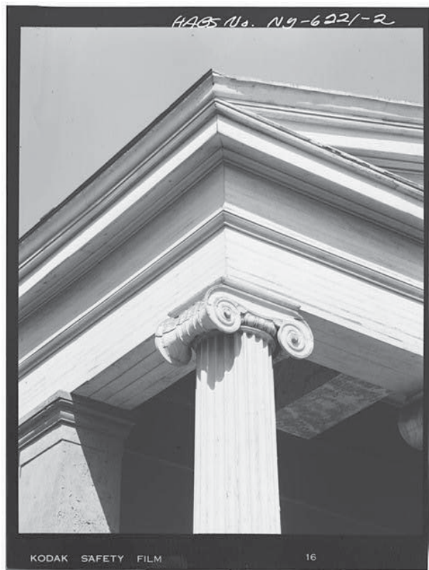
Figures 28, 29 and 30. The design of the volutes is based on engravings from Stuart and Revett's Antiquities of Athens (see History). The HABS photograph above shows their graceful relationship to the column shaft. Right, detail of volute, and below, sundry capital pieces in the storage room.
