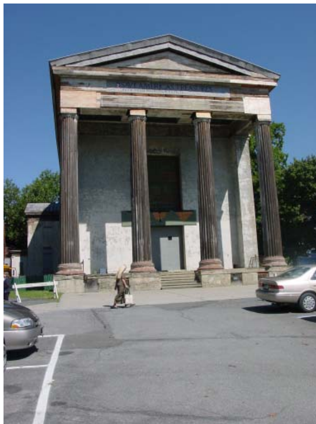
Figure 24. Spalled stucco on east facade between window W23 and W24; note plywood covering portions of entablature.
