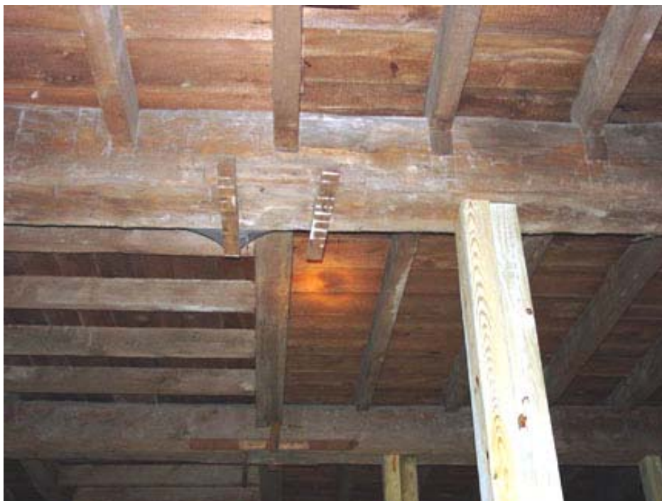
Figure 46. Framing of main level viewed from basement. Note the short joists beneath the aisles to the left of the photograph. The aisles were 4" below the pew areas according to Davis' specifications. The furring strips indicate the original position of the columns.
