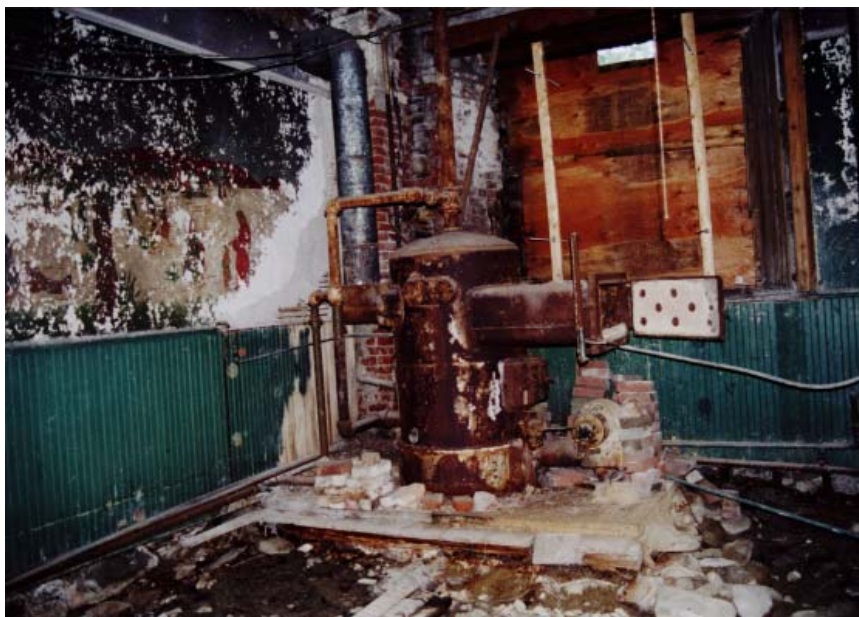
Figure 73. Defunct furnace in west School Room.
