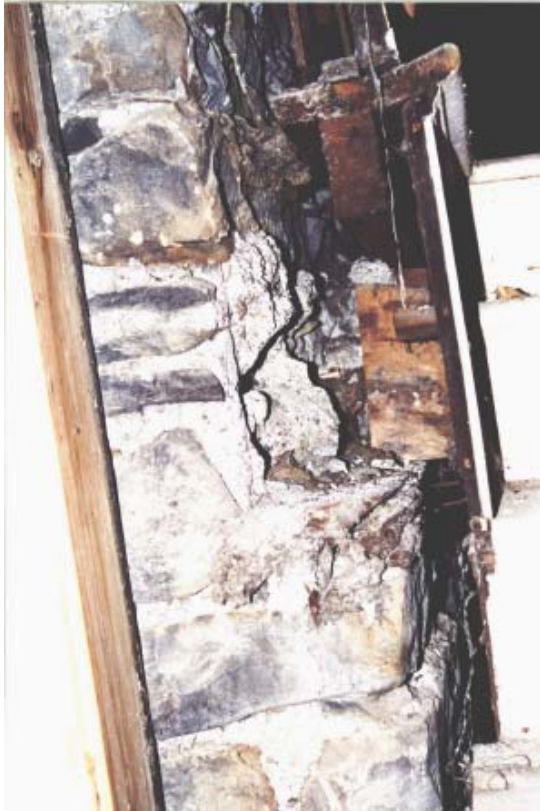
Figure 70. Ledge at west wall supporting gallery framing. The rubble stone masonry walls step in 6" twice over their height, once at the basement level and once at the Gallery level. The Gallery is tipping away from the wall. Its stabilization is a priority.
