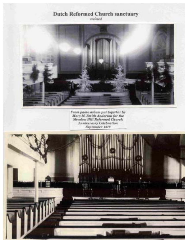
Figure 62. Historical photographs of Nave, north elevation, illustrate the placement of the organ after 1894.
