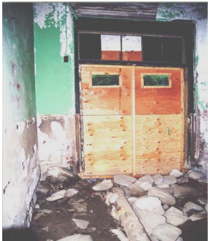
Figure 45. The door opening at west wall of Sessions Room gives clues to the size and configuration of the historic doors installed in 1867. The transom lights are similar to those in the Vestibule on the main floor. The doors once opened onto a passageway between the east and west Areaways that gave access to both the School Rooms and the Sessions Room.
