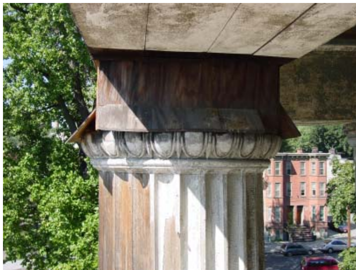
Figures 26 and 27. Base, capital and shaft of Ionic columns. Note the traces of paint on the protected side of the column. The sandstone base was at one time painted, however, it is not known if they were originally painted. The remaining carved wood volutes are stored in the building interior. A master restoration wood carver will explore various alternatives for the restoration of the wood elements of the columns. Prescriptions should be developed for the conservation of the sandstone bases as well.
