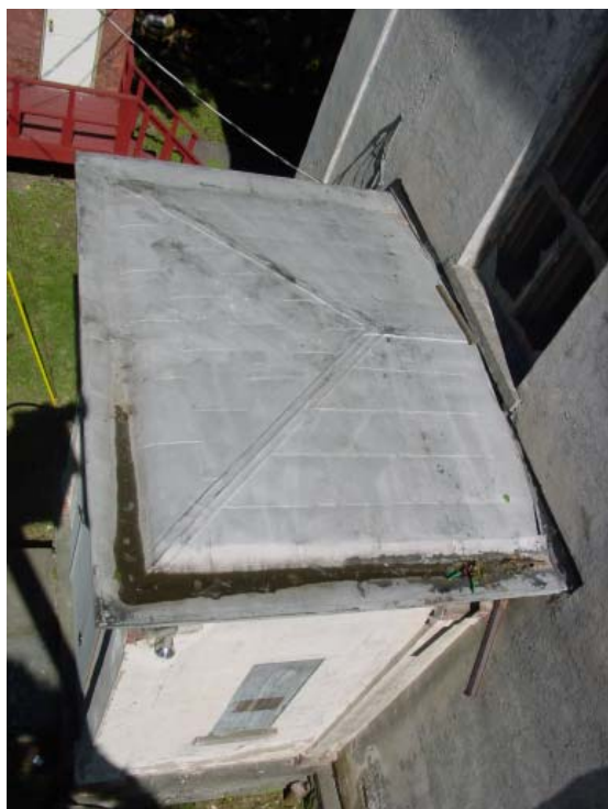
Figures 35 (left) and 36 (above). West entry roof with aluminized coating. Although there is general wear, the roof does not need immediate repair. The roof of the west Transept is a flat seam metal roof very much in need of repair. The roof of the west Transept is standing seam metal. The pans have lost their protective coating and show signs of deterioration which may lead to leaks affecting the interior of the building.
