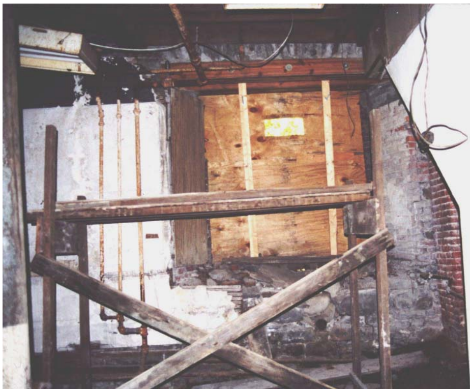
Figure 48. The shored window at east wall of East School room is representative of the stabilization efforts undertaken by the National Parks Service in 2002.
