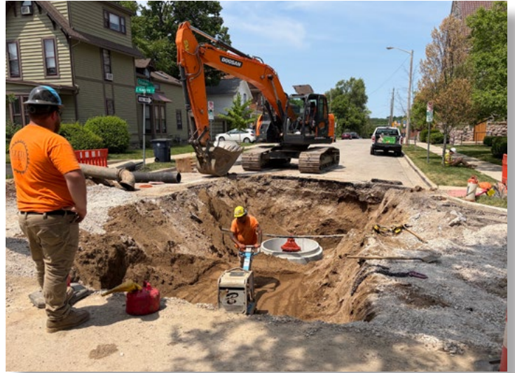
CONNECTING WATER MAIN TO HOUSES
