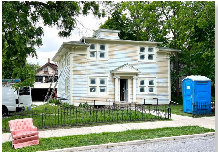
NEW PAINT JOB UNDERWAY
