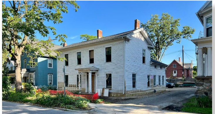
511 E. ANN – DURING RENOVATION
