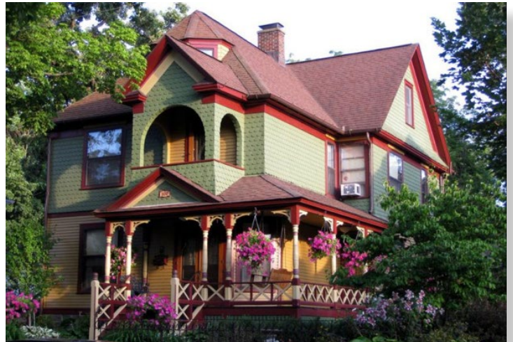
FRONT VIEW OF COMPLETED HOUSE PAINTING AND PORCH REPAIR
