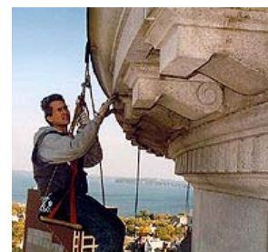
Wisconsin State Capitol. Photo: Wiss, Janney, Elstner Associates, Inc.
