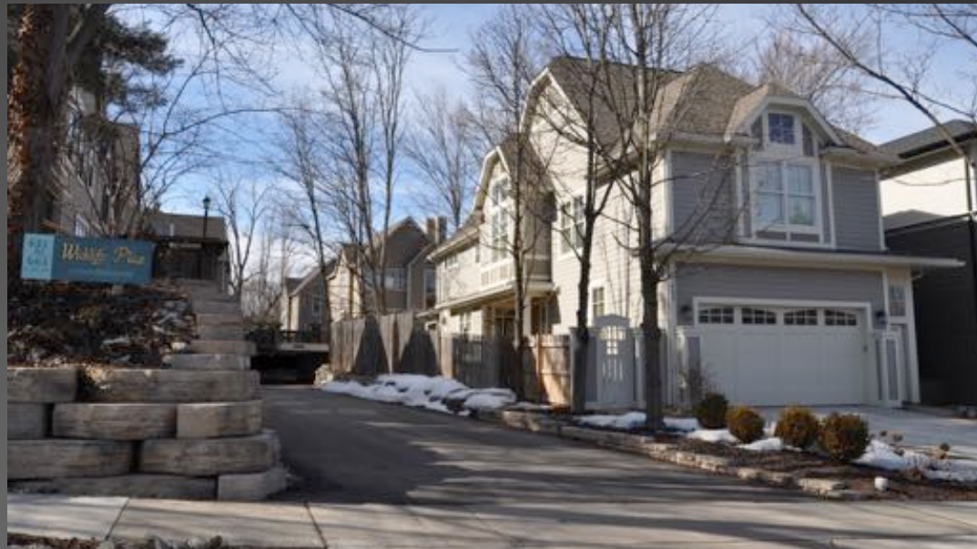
Wickliffe Place Condominiums
