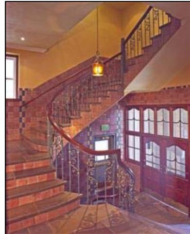
Restoration of historically significant building features included the main entrance doors and plaques, the mica shade light fixtures and Pewabic wall tiles in the main hall, and the light fixtures and verdigris bronze handrail finish in the stairwell and lower level.
