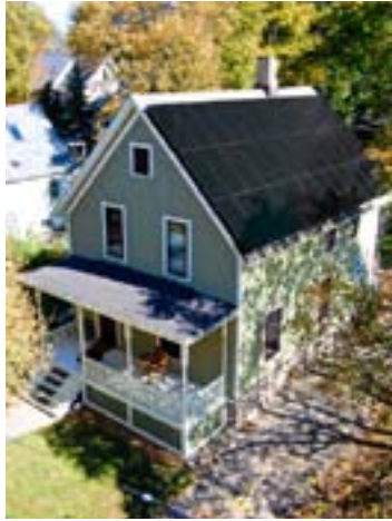
Solar panels cover the entire southern exposure of the Grocuff roof.
