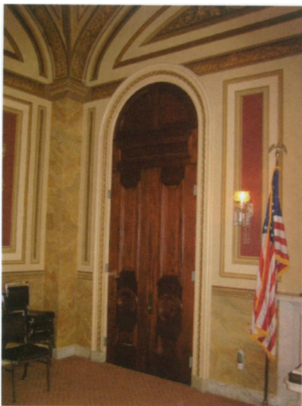
Fig. 2. Cast-iron enframement of doorway in Senate Room S-211, the Lyndon Baines Johnson Room, at the Capitol. All photographs by the author unless otherwise noted.
