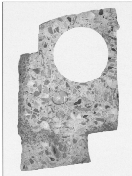
Fig. 4. Cross-section of regula piece with mutule. The hole is where a core sample was taken for laboratory testing. The step-graded buff mix is visible in the section, as is the steel bar reinforcing. A dark line around the steel bar indicates slight corrosion, also indicated by hairline cracks radiating outward from the bar. Courtesy of Wiss, Janney, Elstner Associates, Inc.
