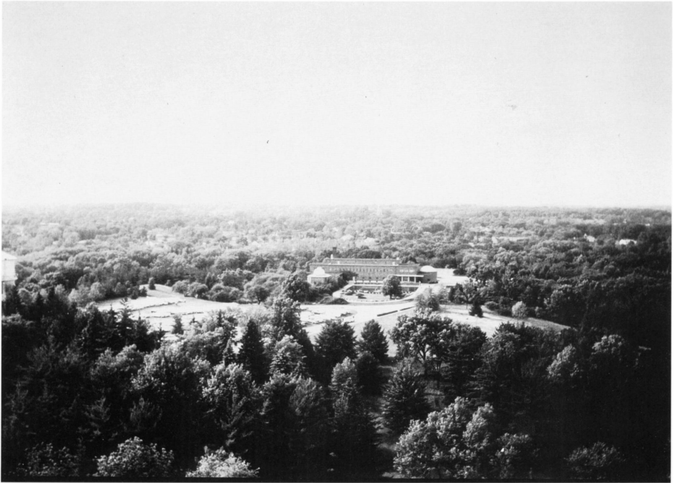
Fig. 2. The first landscape, aerial view from 1958 of Cranbrook Institute of Science, built 1930, with established tree cover (FD 82.44). (Cranbrook Educational Community Archives)
