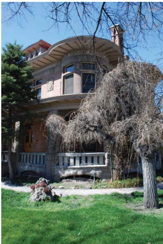
5. View of south-east stone spigot and weeping mulberry tree.
