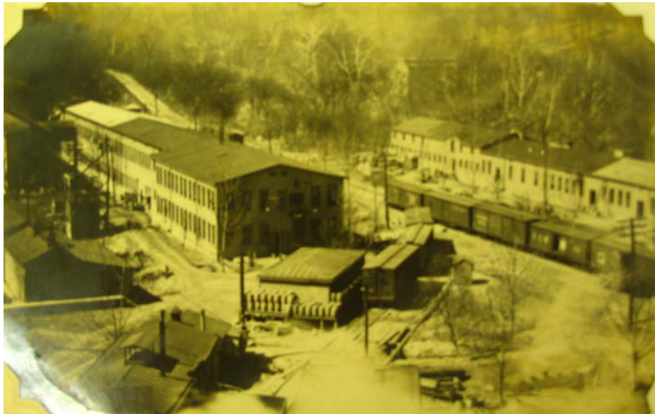
Figure 14. Early view of Peters Cartridge Company, looking southwest
