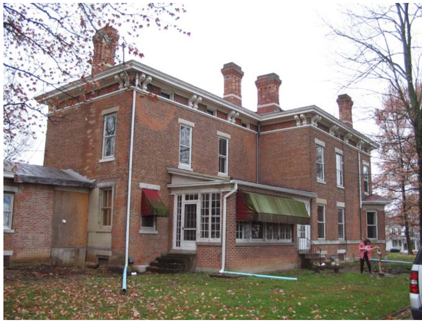
Photo 3. West and north elevations, looking southeast
