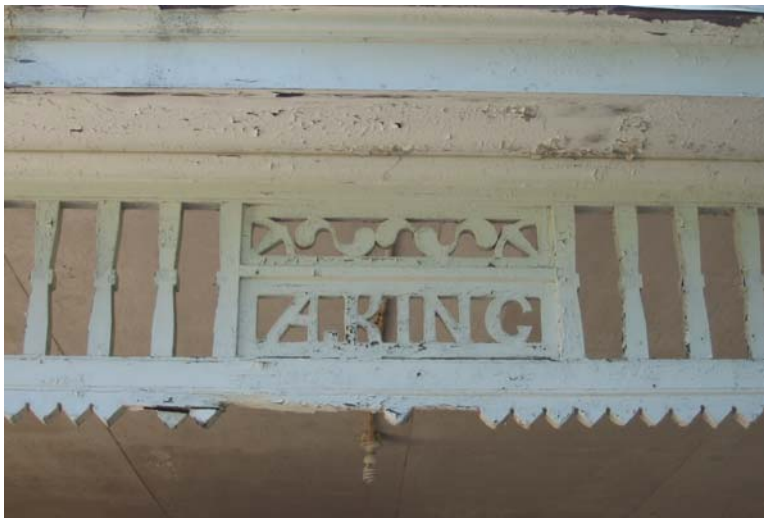
Photo 13. Carriage House, south porch detail
