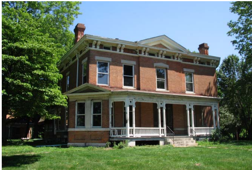
Photo 1. Front elevation, looking north
