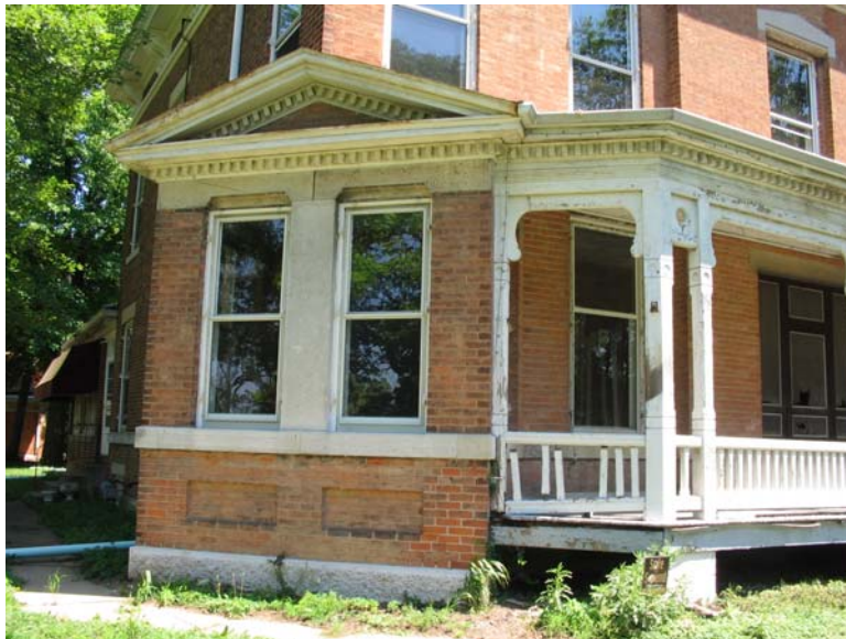
Photo 2. Southwest corner bay
