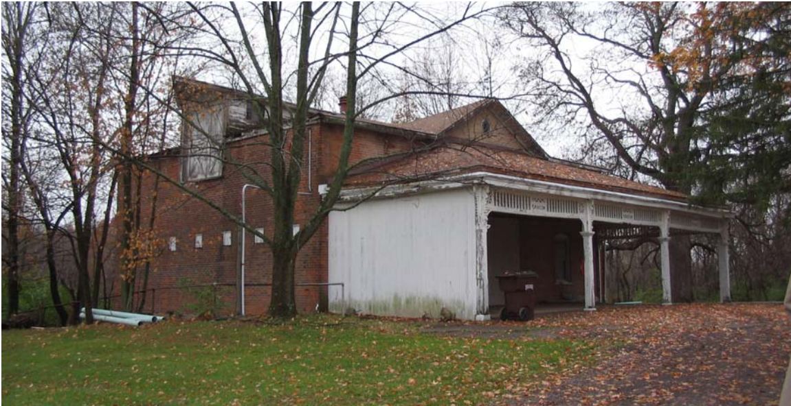
Photo 12. Carriage House, south and west elevations
