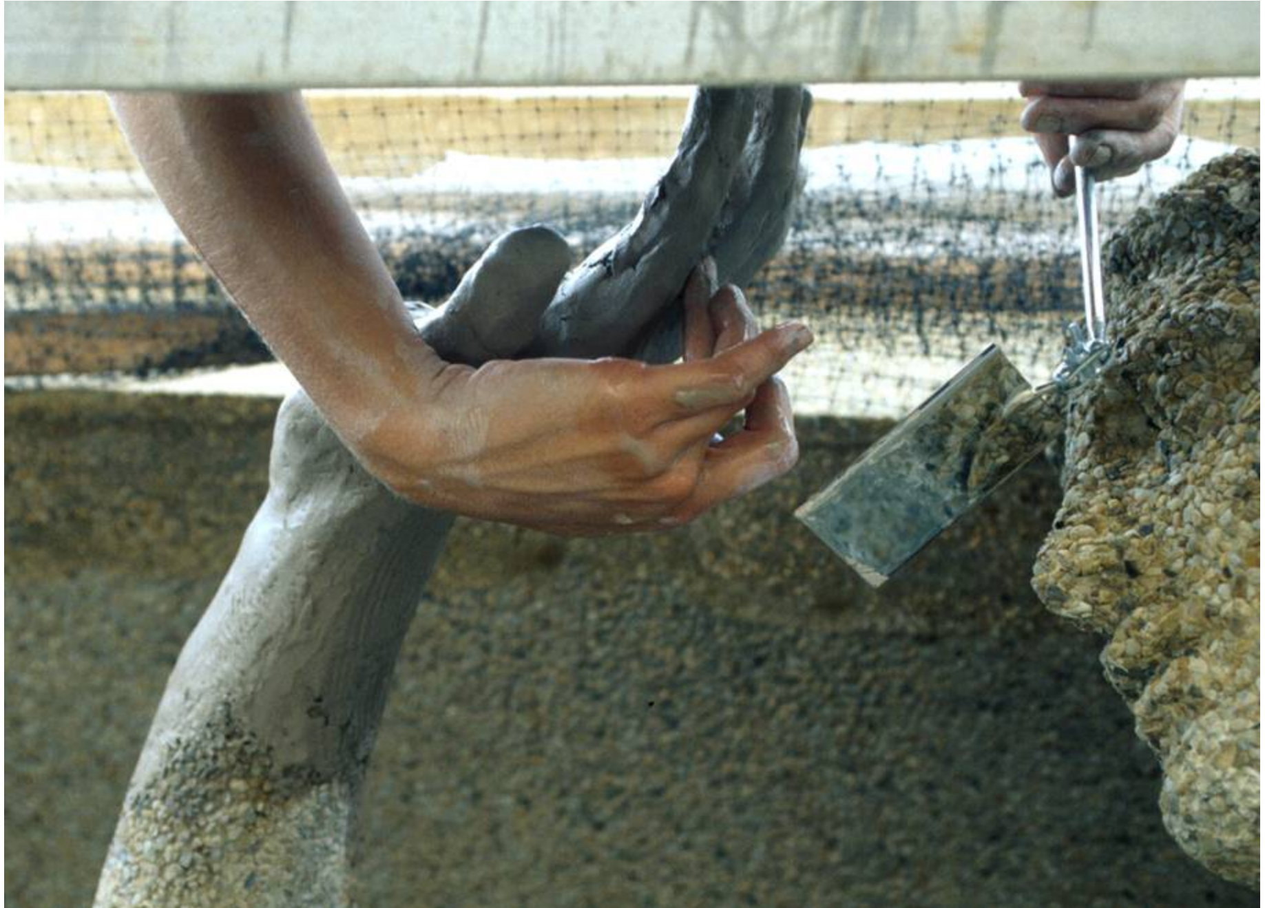
Artists worked from scaffolding to model large and small details in situ.
