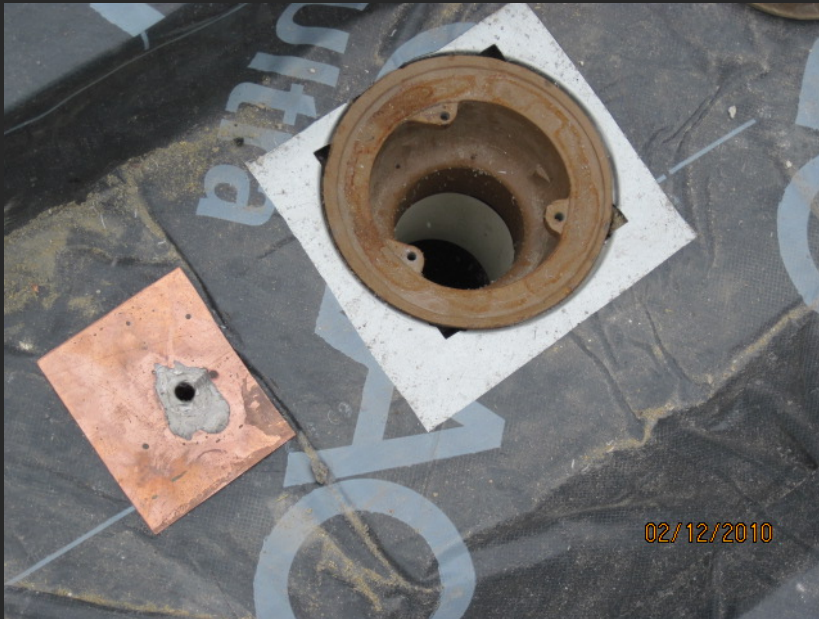
Drain under the Copper
