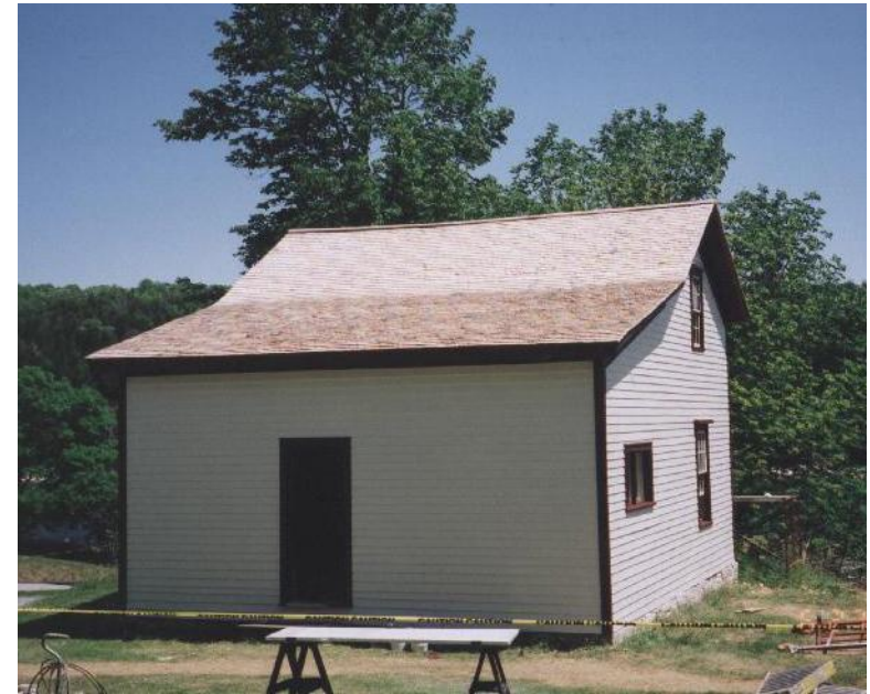
Fayette State Park, Bldg. No. 3 – New cedar shingle roof
