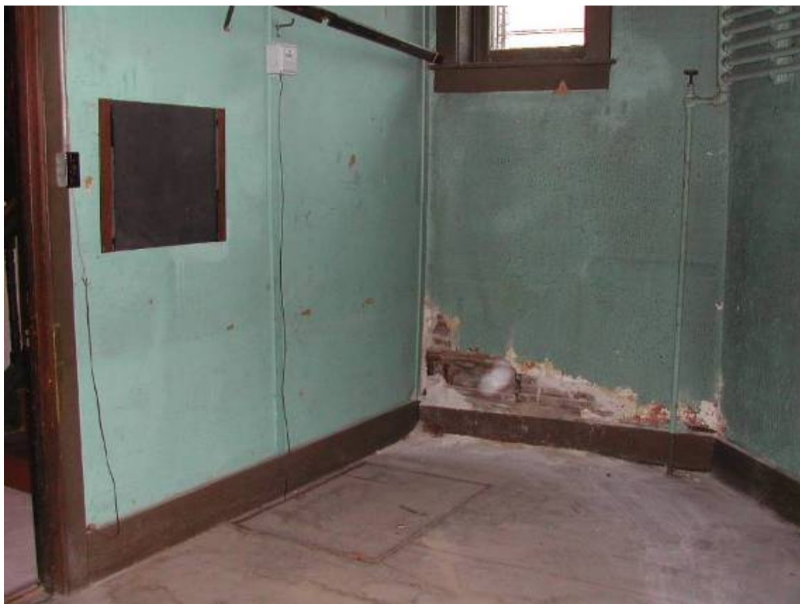
Gardner Museum of Architecture & Design Quincy, Illinois Basement under Entrance
