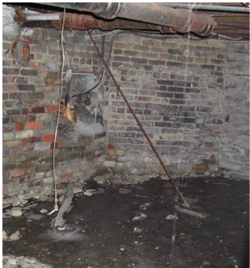
Pere Marquette Depot Bay City, Michigan Basement/Crawl Space
