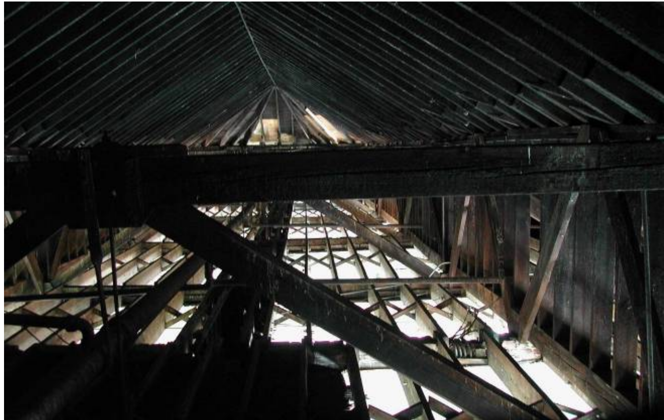
Pere Marquette Depot Bay City, Michigan Attic Structure
