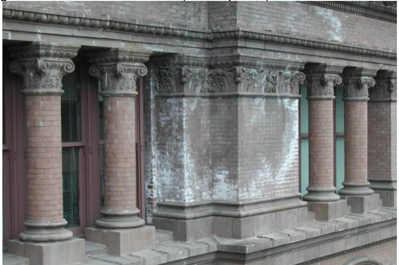
Milwaukee City Hall Milwaukee, Wisconsin 8 th floor, exterior masonry
