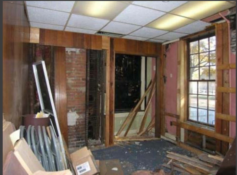
Paint sampling and "Selective Demolition" Miller House, Springfield, Illinois
