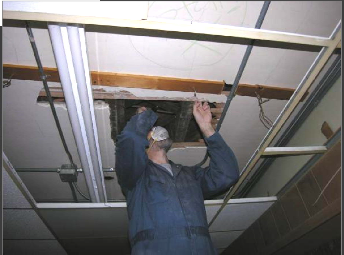
Miller House, Springfield, IL – Conditions Survey for HSR
