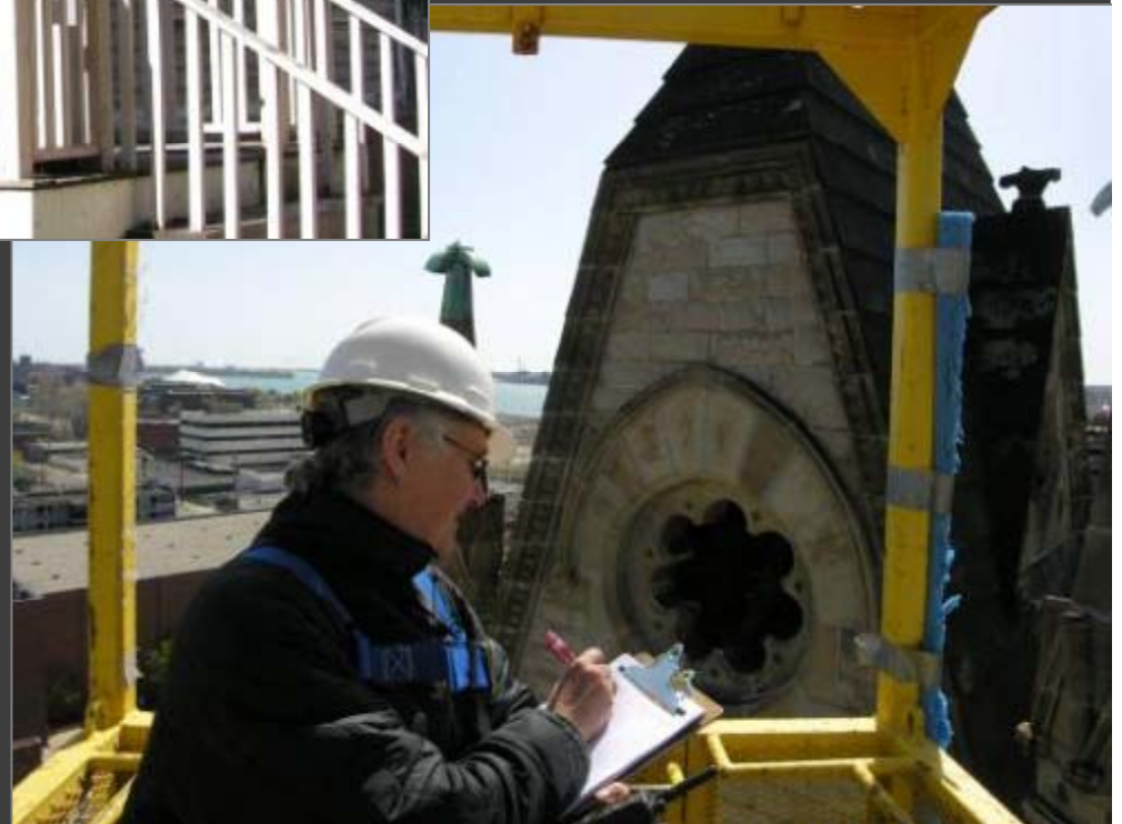
Christ Church Detroit – Masonry Conditions Survey
