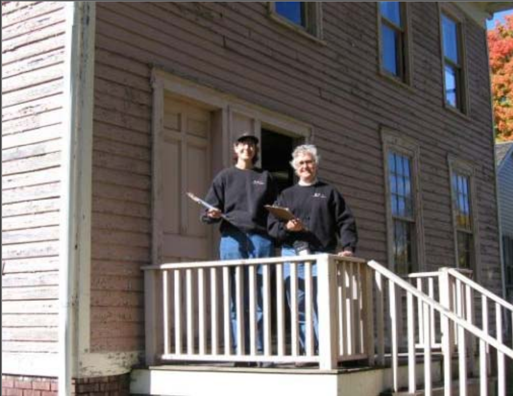
Miller House, Springfield, IL – Conditions Survey for HSR
