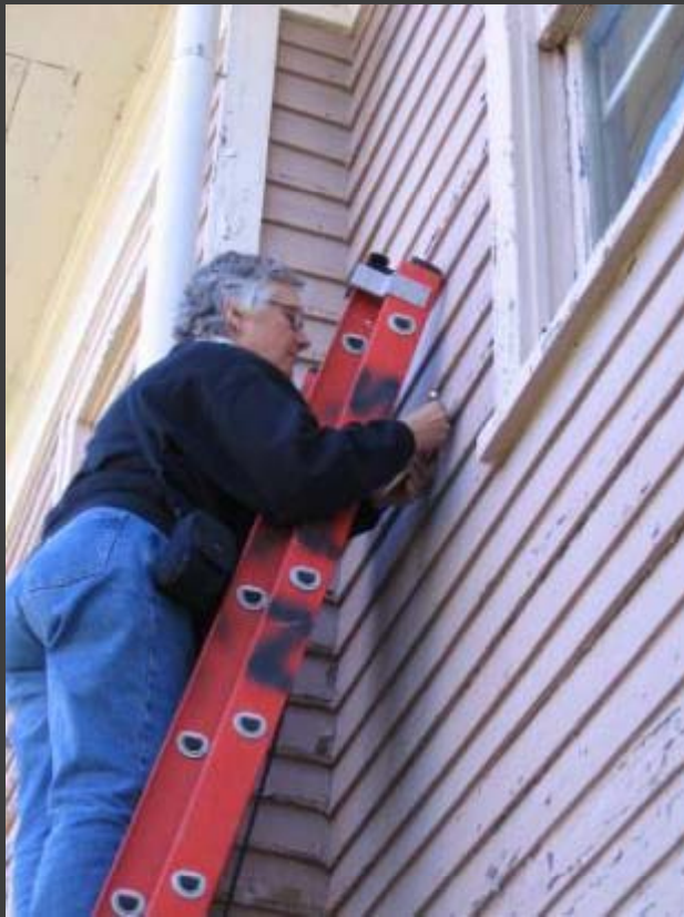
Paint sampling and "Selective Demolition" Miller House, Springfield, Illinois
