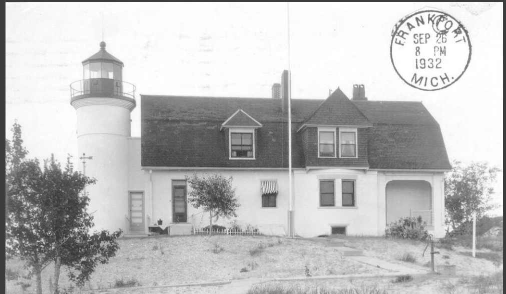
Before and After Restoration Point Betsie
