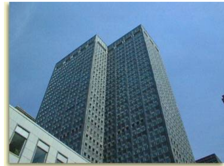
Alcoa Building, 1953, Pittsburgh
